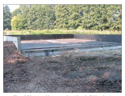
Photo 5.5 Impermeable manure plate (photo by P. Nawalany)
