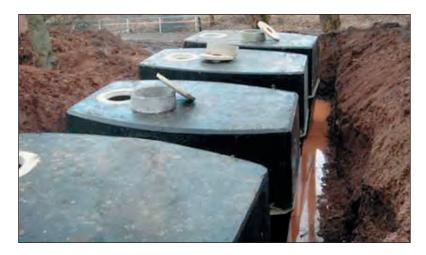
Photo 6.1 Tanks for liquid manure and slurry (photo by P. Nawalany)
